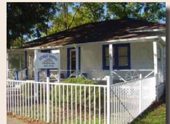
CATHOLIC CHARITIES OFFICE AND COMMUNITY CENTER AT 21257 CALISTOGA STREET, MIDDLETOWN
