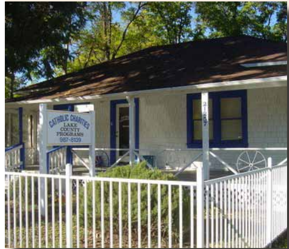
CATHOLIC CHARITIES NEW MIDDLETOWN OFFICE AT 21257 CALISTOGA STREET
